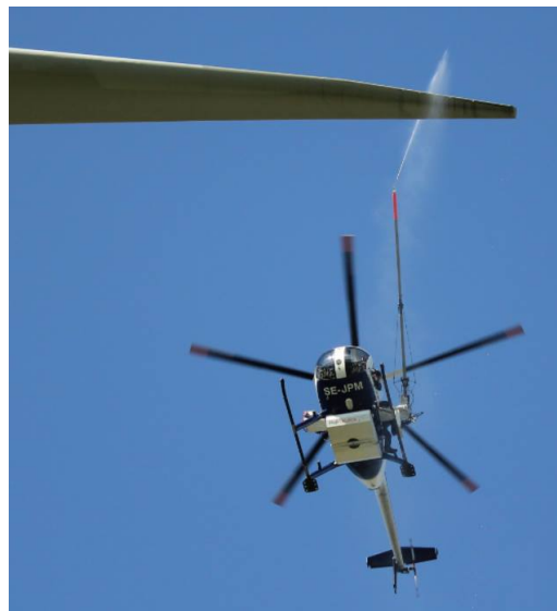
Figure 9: Helitechnics® cleaning wind turbine blade with water canon.
